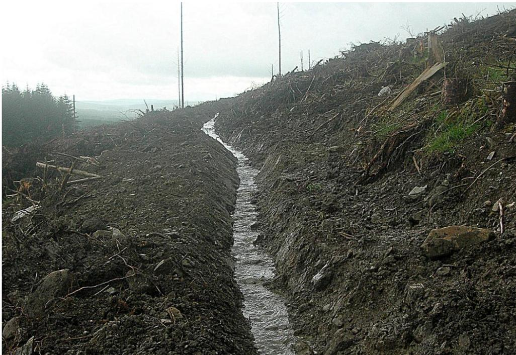
**Figure 2-19: Newly constructed drainage ditch.**
