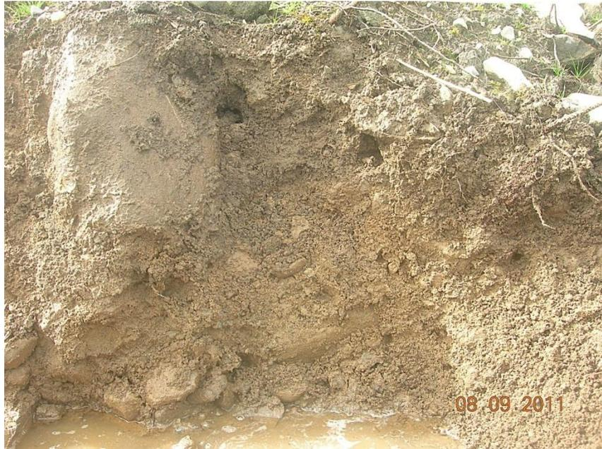
**Figure 5-6: Example of exposed face of inspection trench DS1 showing irregular boundary between dark humic disturbed soil and underlying stonier material**
