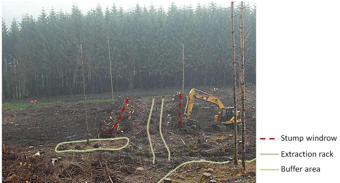
**Figure 2-31: Layout of destumping operations, June 2011.**
