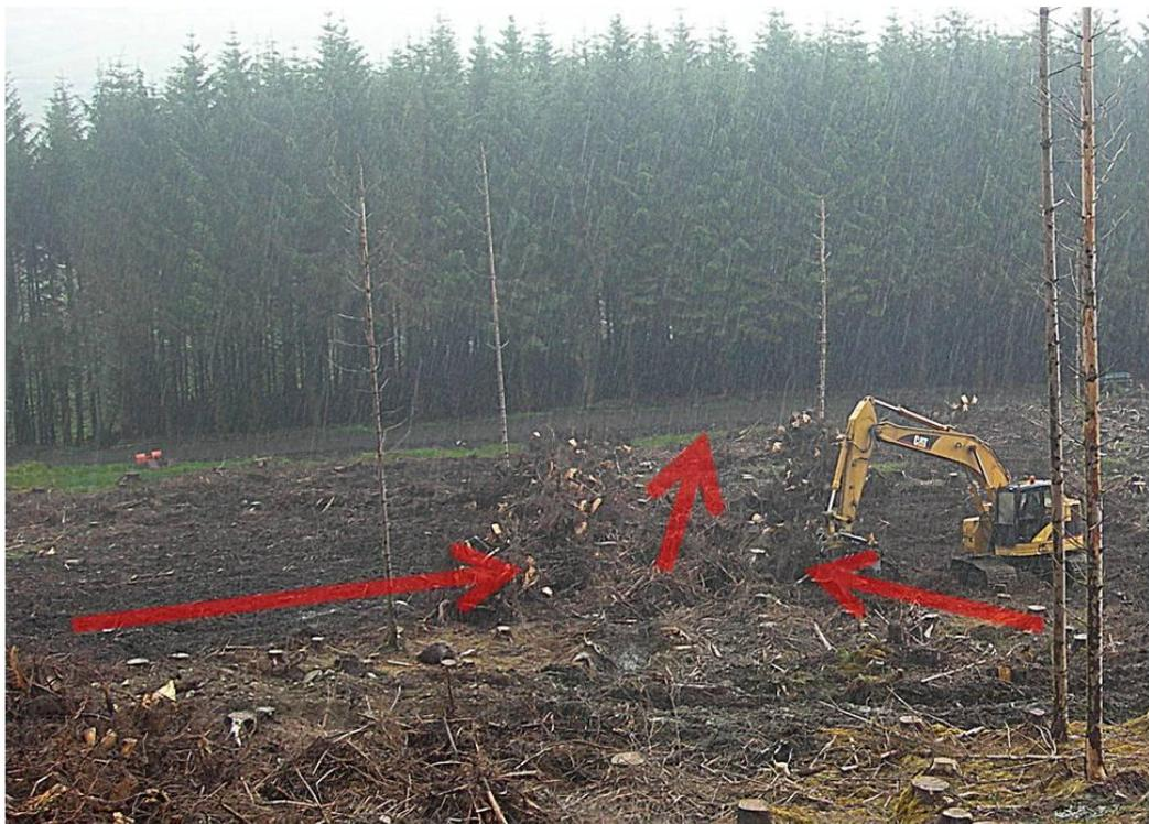
**Figure 5-35: Destumping zone layout indicating movement of stumps to windrows and subsequent transport to roadside by forwarder along existing extraction route.**
