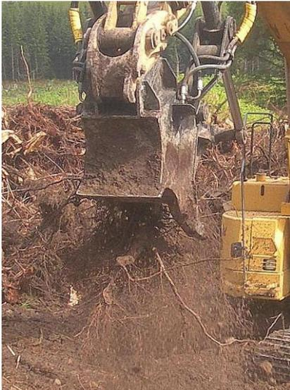
**Figure 6-1: Soil falling to ground as stump is lifted and crushed.**
