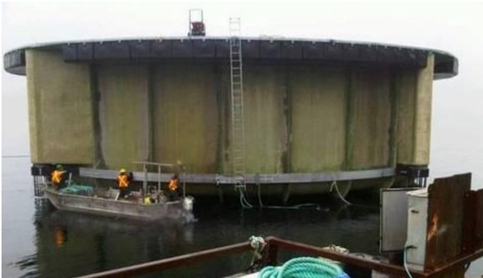
Figure 10: An Agrimarine floating closed containment system being prepared for installation 46
