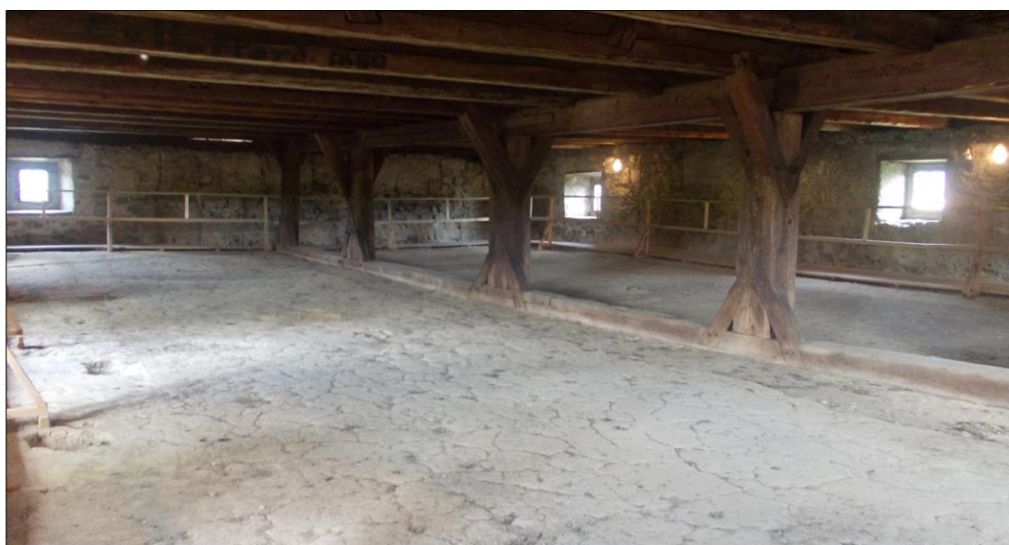
Fig. 4.15. Beaten mud floor on the top level of Siedlecin Tower, Lower Silesia, Poland. This was laid above the ceiling of the underlying level, where it is visible through the timbers, and provided good insulation for the Great Hall below.
