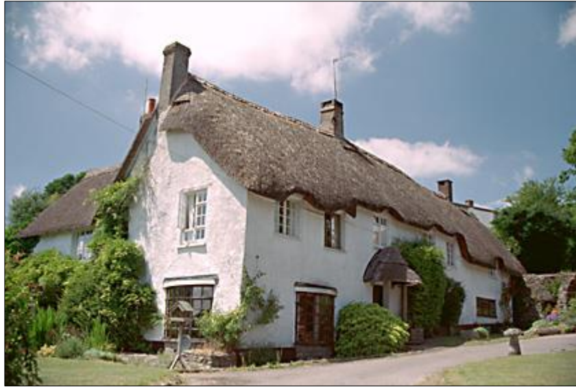
Fig. 3.2. Bridford Barton, Bridford, Devon. Cob and stone built farmhouse of early to mid-fourteenth century origin. (Photo credit: © Mrs Jean M. King C.P.A.G.B.).
