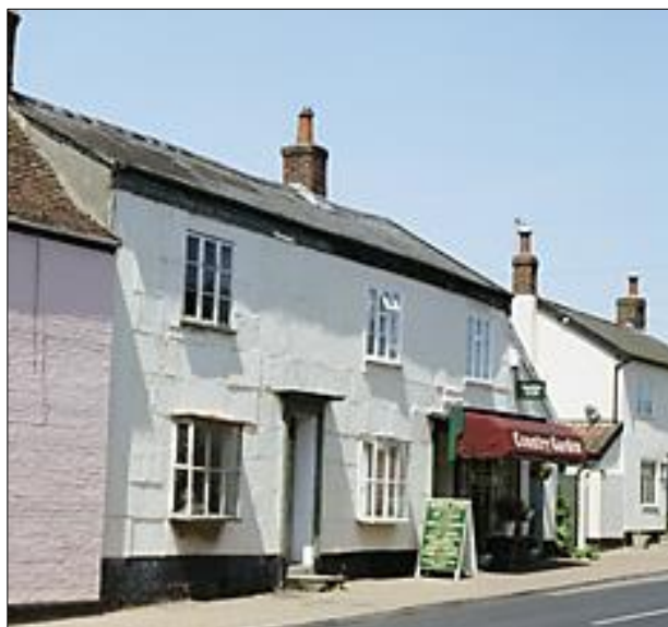
Fig. 3.4. Hilltop House, Botesdale, Suffolk. A prime example of early nineteenth century clay lump construction. (Photo credit: © Prof John N. Buxton).
