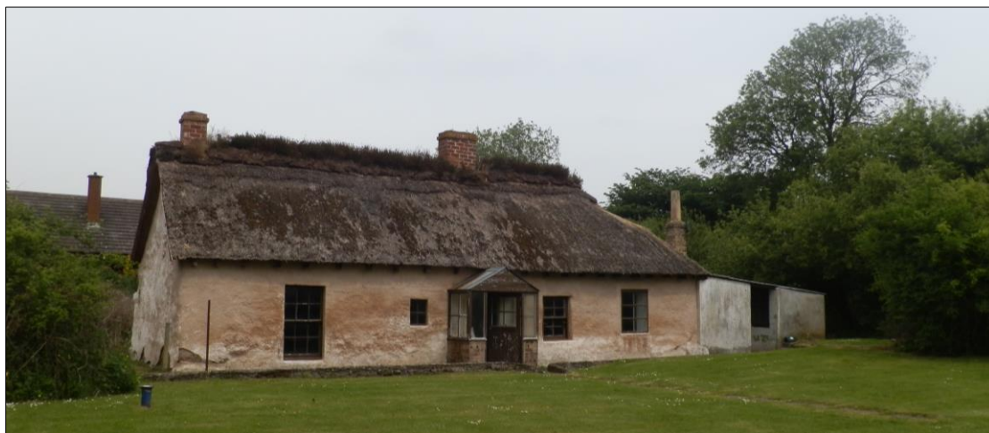
Fig. 7.5. Water marks on the walls reflect the rise of water from the ground and during previous flooding events. Feilden (2003) suggests that the height of wetness at the surface of masonry walls reflects the levels to which critical water content has been reached internally.
