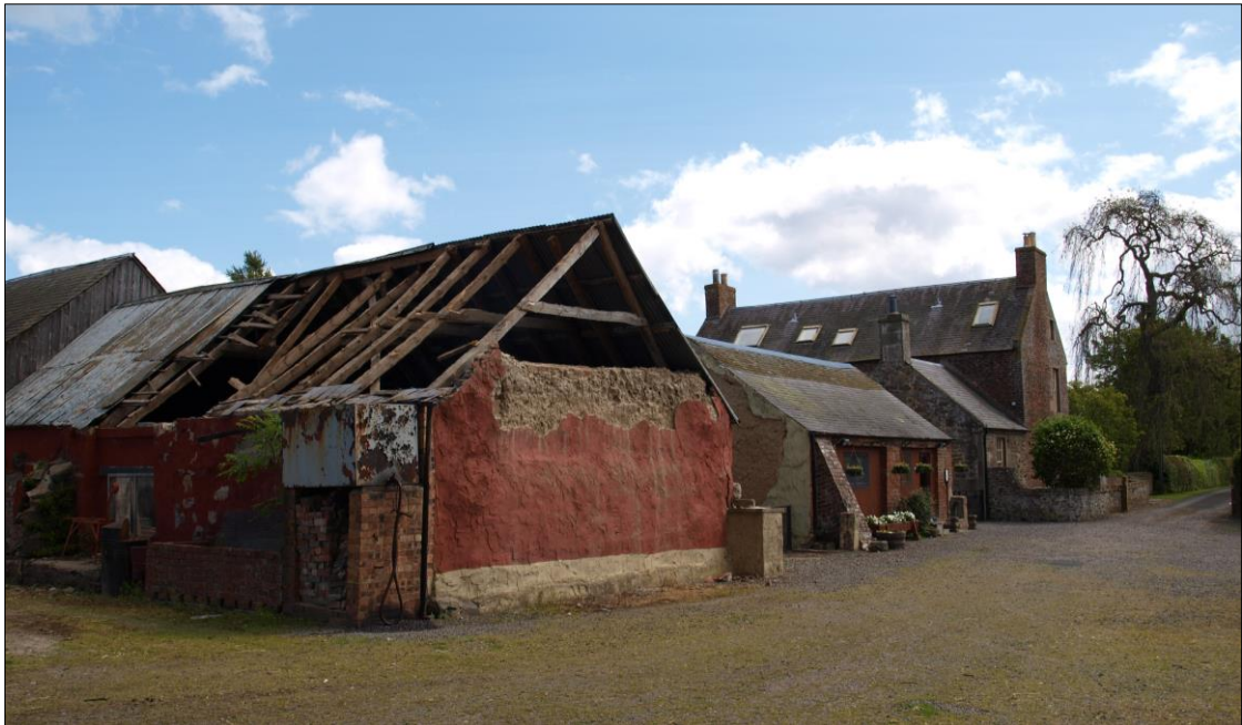
Fig. 7.14. The cement render has failed and is gradually being shed from the walls of the barn and cattery. Although this seems to be taking place without causing excessive damage to the underlying fabric, the brick gable of the barn is now completely lost as a consequence of the deterioration caused. High winds in 2011 resulted in the loss of the corrugated iron roof from the barn and left it in a precarious state.
