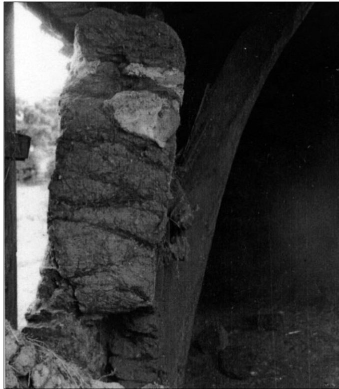
Fig. 4.6. Barn at Prior Linn, Canonbie, Dumfries and Galloway, with layers of straw laid between mudwall lifts. It should be noted that this practice could result in the increased exposure of straw to moisture and therefore decay, thus undermining the strength of the walls (Morton, 2008). (Photo taken by Werner Kissling in 1954 and held by the School of Scottish Studies Archive, University of Edinburgh).
