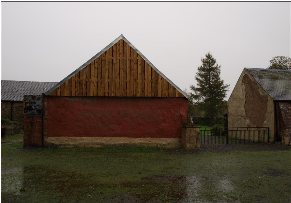
Fig. 7.15. Remedial works to the roof undertaken at the volition of the owners have since ensured the protection of the walls of the barn.
