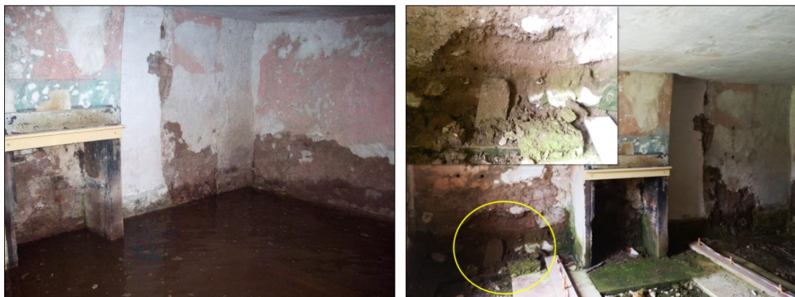
Fig. 7.9a (left). Internal flooding in the west room of the Schoolhouse, February 2011. Fig. 7.9b (right). July 2013: the impacts of repeated flooding are most prominently displayed at the internal side of the west gable wall, where repair blocks are being lost from the body of the mudwall.
