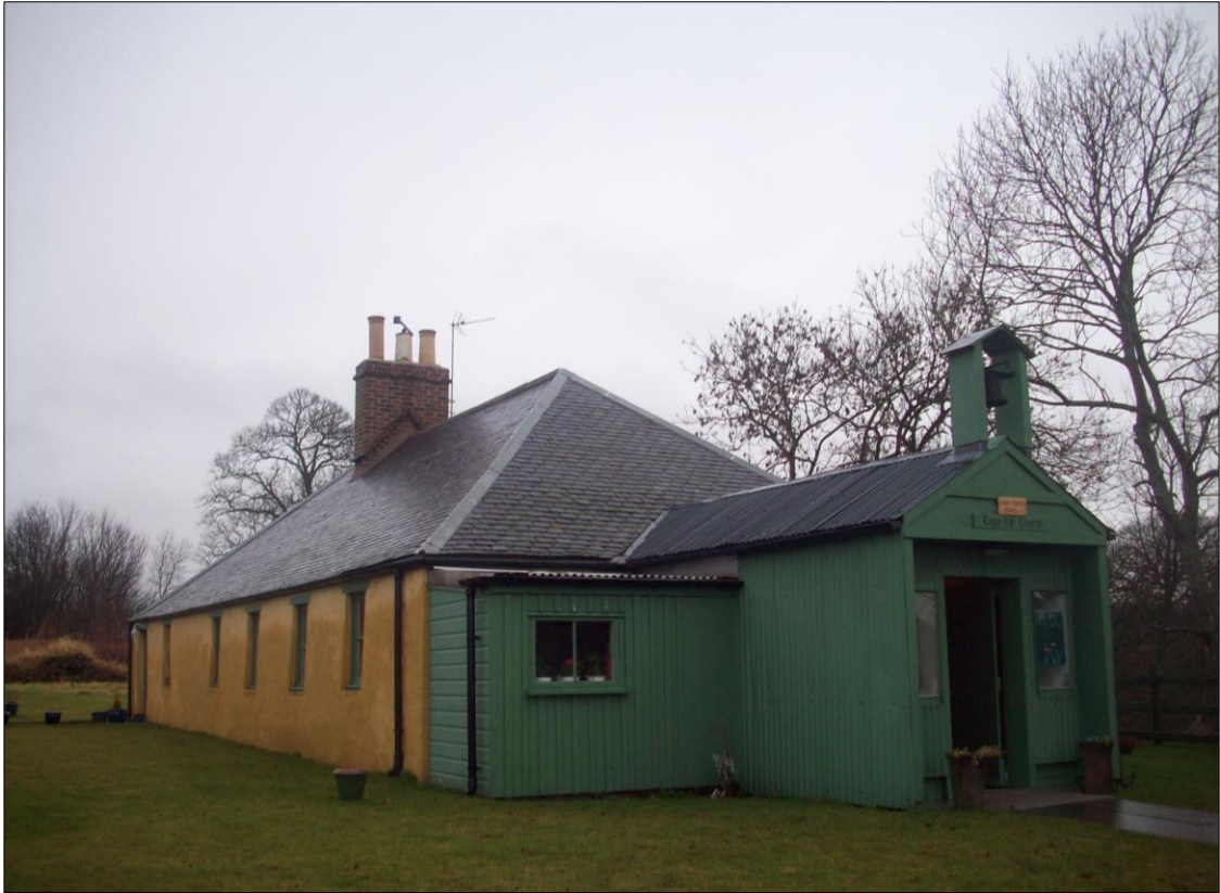
Fig. 4.3. Restored schoolhouse, Logie, Angus. Built in the first part of the nineteenth century, the building was acquired by the National Trust for Scotland (NTS) in 1995 following its abandonment in 1990 and gained an A listing status. The application of cement render in the 1970s had accelerated the deterioration of the mudwalls and the building required major stabilisation and reconstruction. The Schoolhouse was taken on by the NTS Little House Improvement Scheme in 2005, with renovation works commencing in 2007 and culminating in 2008 (Romankiewicz, 2005; Copp, 2009). In 2009 the building was awarded the Europa Nostra Prize, the European Union Prize for Cultural Heritage.
