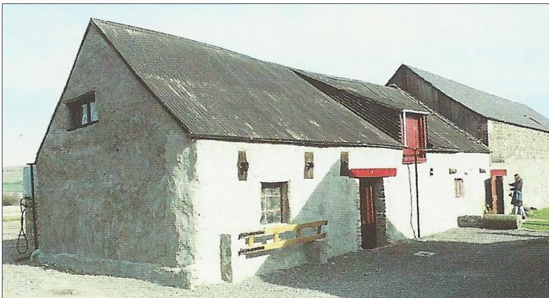
Fig. 7.13. The barn at Flatfield following the application of cement render in the 1970s. (Image taken from McCann, Clay and Cob Buildings [2004]).
