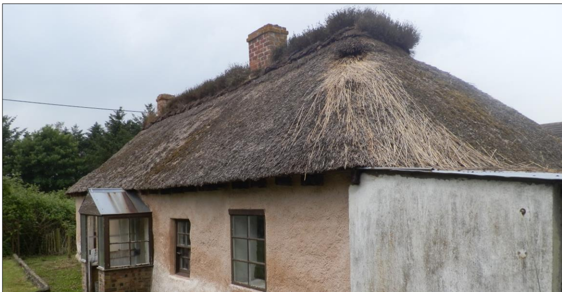
Fig. 7.8. Evidence of thatch deterioration, presumably as a result of bird activity. Such processes can have corollary implications in terms of water ingress.
