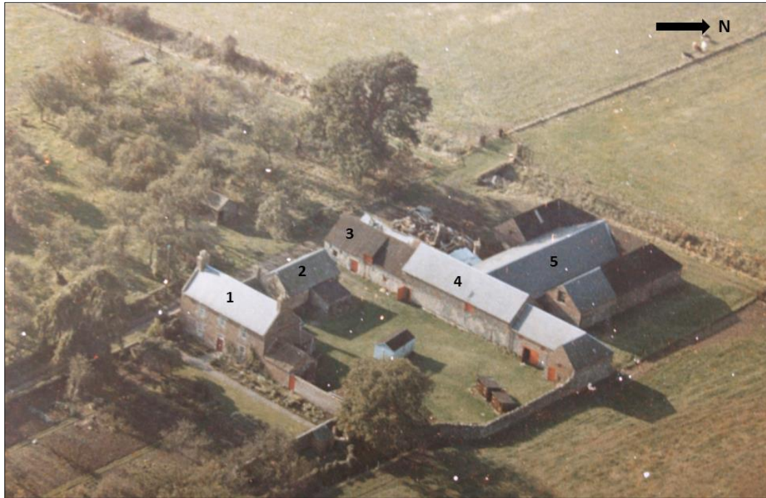
Fig. 7.12. During the 1970s cement render was applied to the exterior surfaces of all of the mass earth outbuildings with the ill-advised intention of protecting the mass earth walls. The numeric labels applied to the aerial photograph donate the following: 1. The farmhouse, dated 1785, built with bricks fired on-site in clamp kilns; 2. Detached mass earth outbuilding, originally one and-a-half stories and possibly used as a dwelling. The structure now functions as a cattery; 3. Mass earth storage shed/barn of one and-a-half stories, which has suffered a great deal of damage since the latter-part of the twentieth century. The structure has lost its western brick gable, which perhaps replaced a previously failed extension to the mass earth; 4. Stone-clad claywall extension of the storage shed/barn; 5. Stone-built byres now used as stables. (Image courtesy of Andrew Driver).
