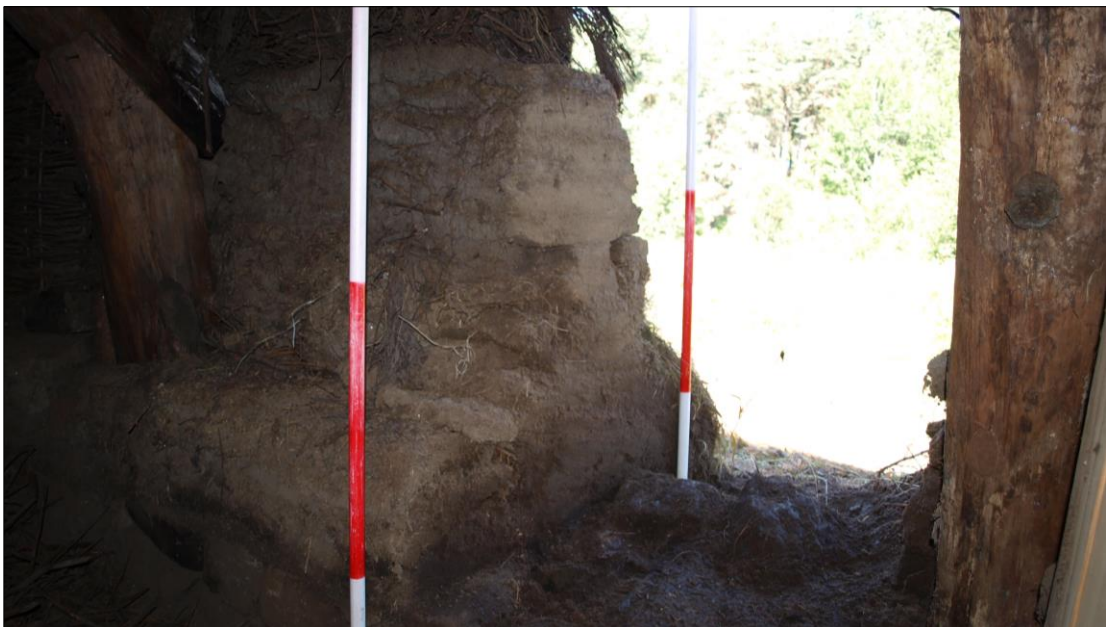
Fig. 4.5. Cross-section through turf wall at the Highland Folk Museum, Newtonmore. (Photo credit: George MacLeod/Dorothy McLaughlin, 2012).
