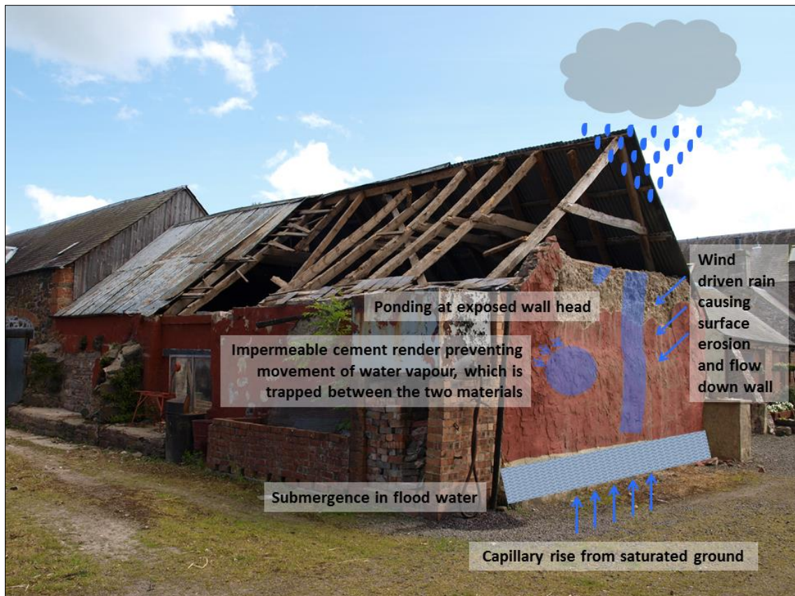
Fig. 5.3. Typical water-ingress issues stemming from inappropriate maintenance and site context problems. As noted, the deterioration of earthen building materials is most commonly related to damage from water ingress, a theme that punctuates the general earth building literature and which clearly has ramifications in relation to projected climate conditions.
