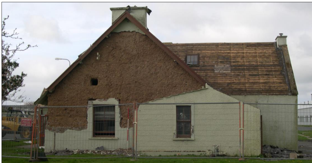
Fig. 11.1. The mudwall farmhouse on MOD land at West Freugh serves as a prime example of the issue of invisibility, with its form and superficial appearance belying the original means of construction and materials and methods employed. Its demolition has meant the loss of a sound mass earth structure that also included marked Baltic timbers and sarked roof construction, which was made possible through the further industrialisation of timber production from c. 1800 (Historic Scotland, 2006). (Image courtesy of Stranraer Museum).
