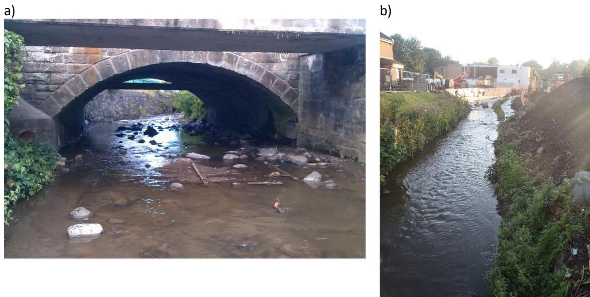
Fig 4.3 Photo of a) failed sediment stopping net and b) in channel and riparian engineering work upstream of IMP1.
