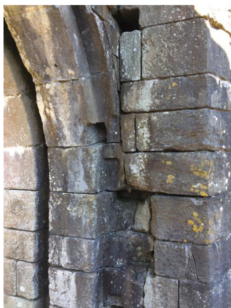
FIGURE 67: PHOTO OF BUTT JOINT OF MAIN ENTRANCEWAY AT LOCH DOON CASTLE; ANTIQUARIAN PLAN OF CASTLE
