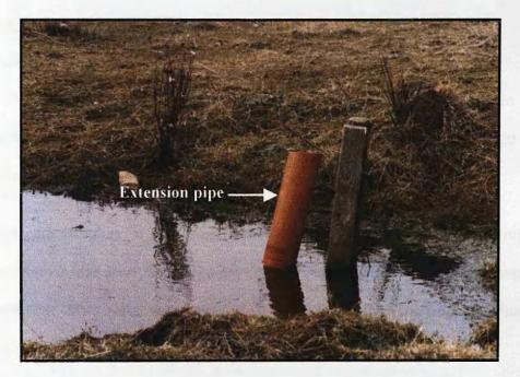
Figure 3a Photograph of HIGH water ditch - showing extension pipe preventing water flow out of ditch.
