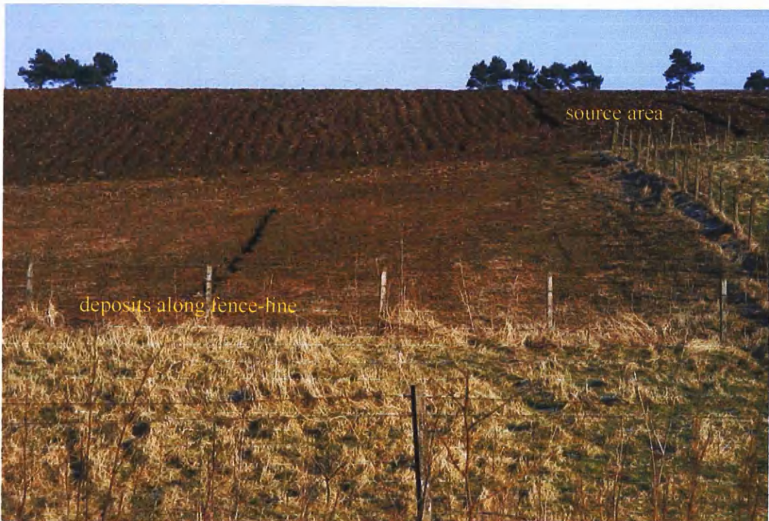
Figure 4.32. View across the Greens Burn to field 2, showing source material being carried down a shallow (approximately 16 cm deep) gully (taken 14 th February 2003).
