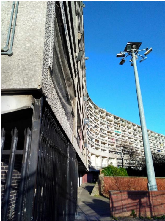
Image 1: Exterior of the House (East-facing/private balcony side), showing the distinctive bend
