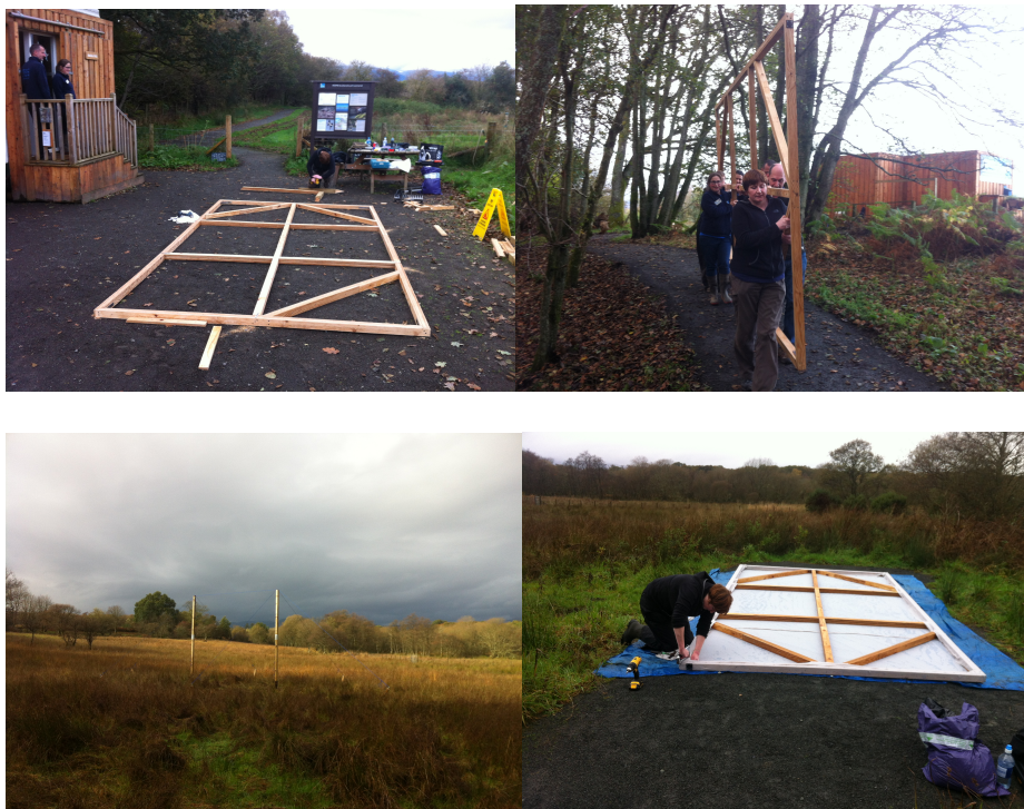
Figure 37. Building the frame and screen for The Essence of Place (2017).
