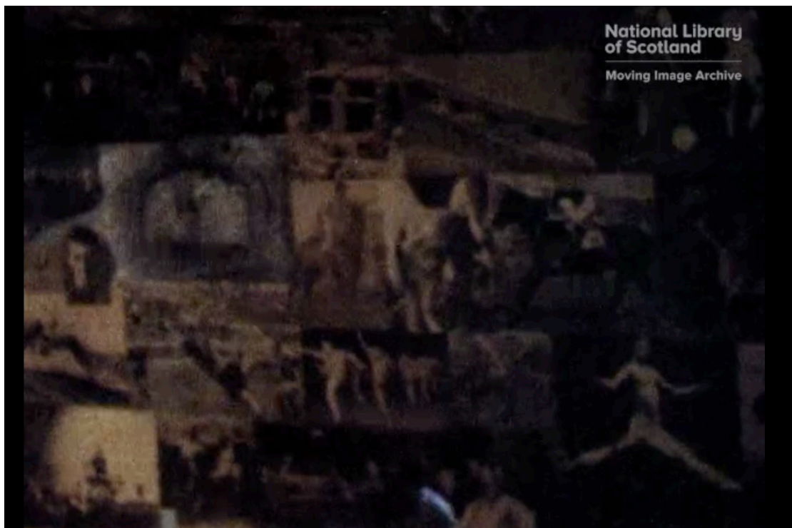
Figure 25. Pictures pasted on Tait’s walls, These Walls (Tait, 1974).
