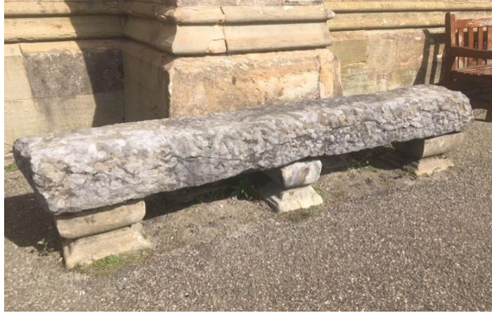
Fig 17: Fossiliferous marble stone c.7' 6" long x 15" broad x 10" deep, on south-side of Abbey Church exterior, removed from the choir high altar remains in 1817 [© David Williams].
