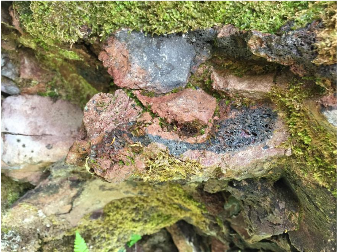
Figure 90: Vitrified and heat damaged rocks at The Torr, Shielfoot.
