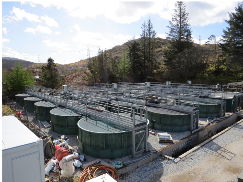
Figure 4-1 Duartmore site, Southside 23 x freshwater tanks
