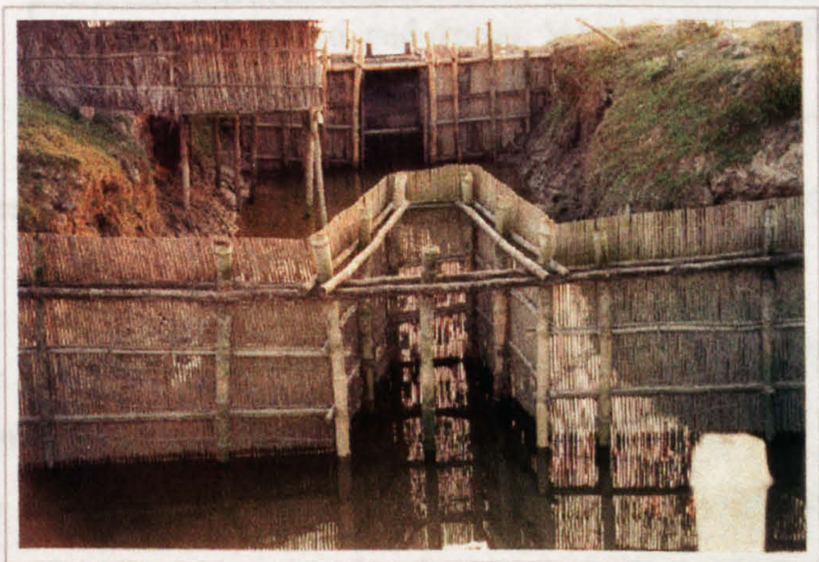
Figure 1.2. Shows the sluice gate built to hold and exchange the water in the shrimp projects in the Khulna region, Bangladesh.
