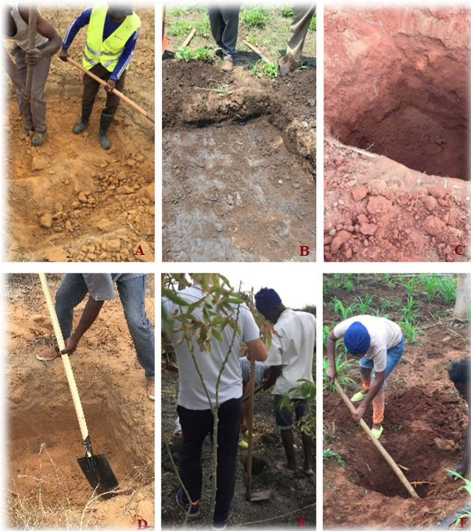
Figure 3. 5: Trench opening. A-Ngongoinga, B-Bailundo, C-Mungo, D-Ramiro, E-Funda, F-Talelo
