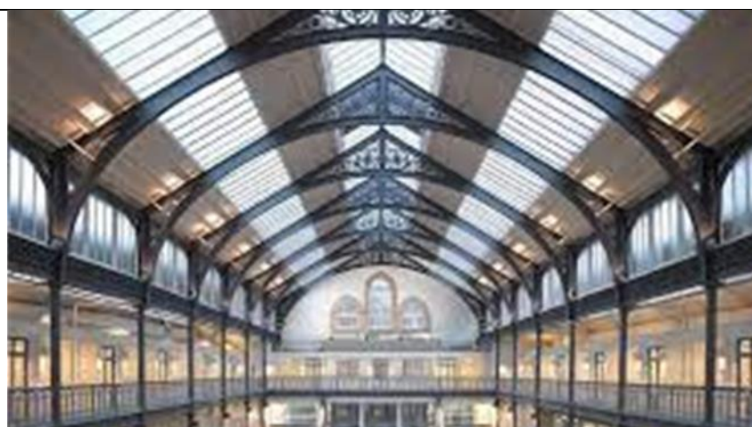
Figure 14 The interior of the Briggait Fishmarket after its restoration
