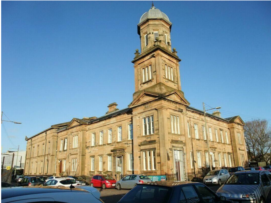
Figure 1: Glasgow Building Preservation Trust, based at the former Wellpark School and Kirkhaven Church, restored by GBPT in 1996
