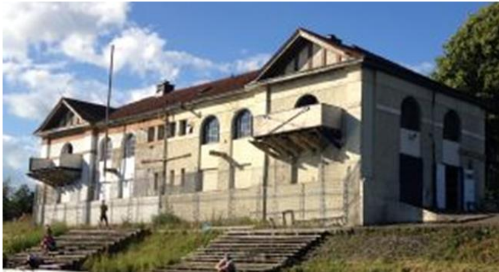
Figure 2. The West Boathouse before its restoration in 2019 seen from the water. Photo by GBPT
