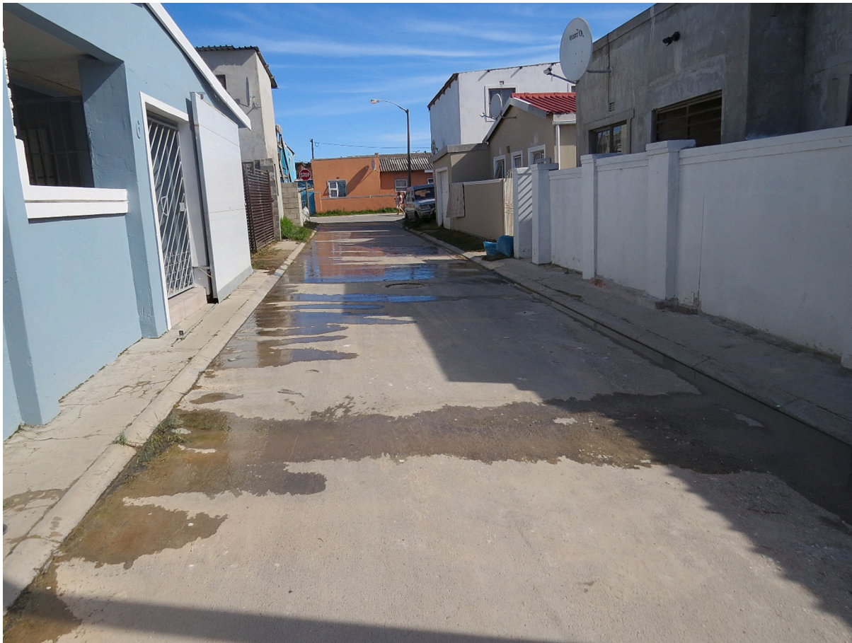
Fig. 3. John's photograph, "Houses on water".
