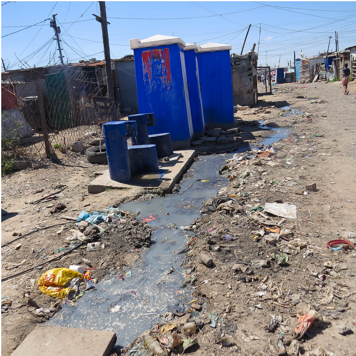
Fig. 5. John's photograph, "Leaking tap".
